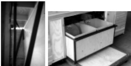
Keg pavilion - details: hinge mechanism (left), keg drawer (right)
