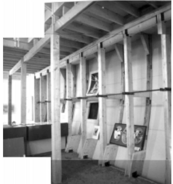
Interior view of "Belly wall" constructed of recycled bow trusses turned vertically
